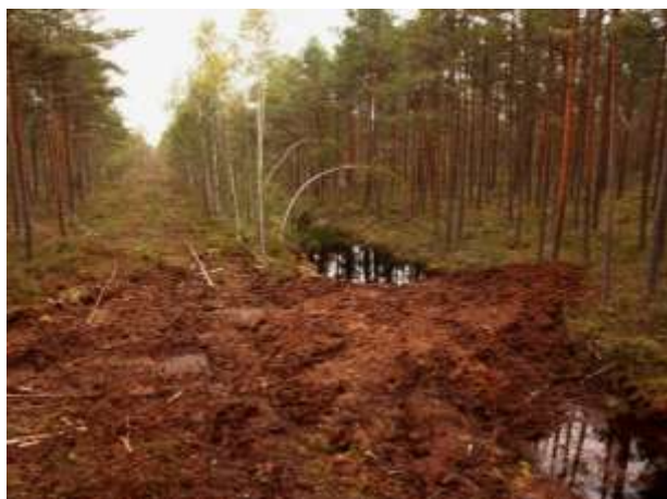
Peat dam on drainage ditch in Rozu Mire.
