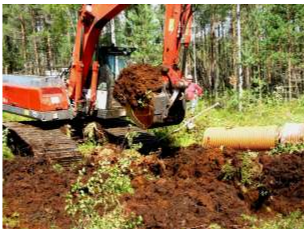
Building of peat dam in Rozu Mire.
