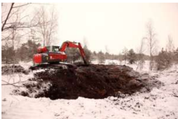
Peat dam on drainage ditch in Melnais Lake Mire.
