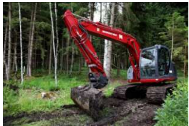
Building dams in the Bavarian LIFE project. Photo: Aivars Slisans
