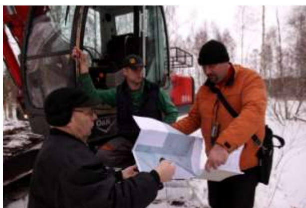
Building of dams in Melnais Lake Mire.
