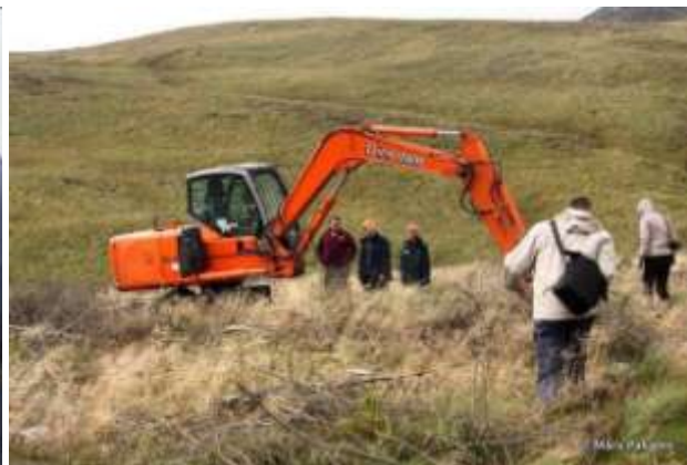
Building of dams in LIFE project site - the blanket bogs in Wales on 01.09.-07.09.2010.
