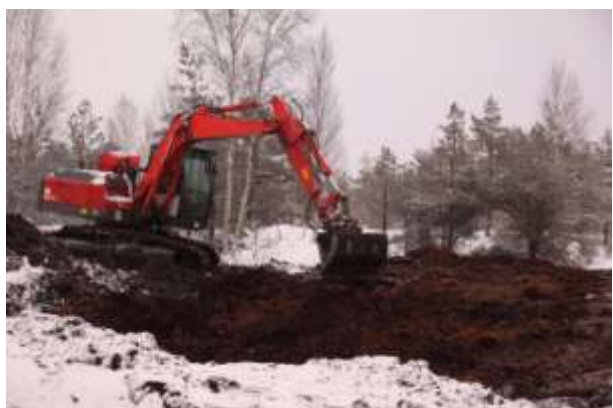
Building of dams in Melnais Lake Mire.
