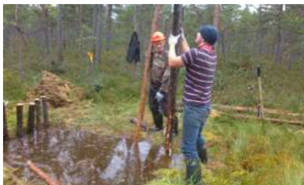
Building of peat/wood dam by hand in Aizkraukle Mire on 03.09.2012.
