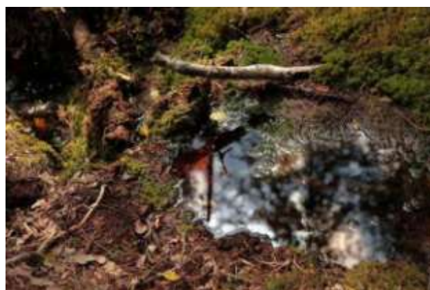
Drainage ditch where dams have to be built in Rožu Mire Nature Reserve.
