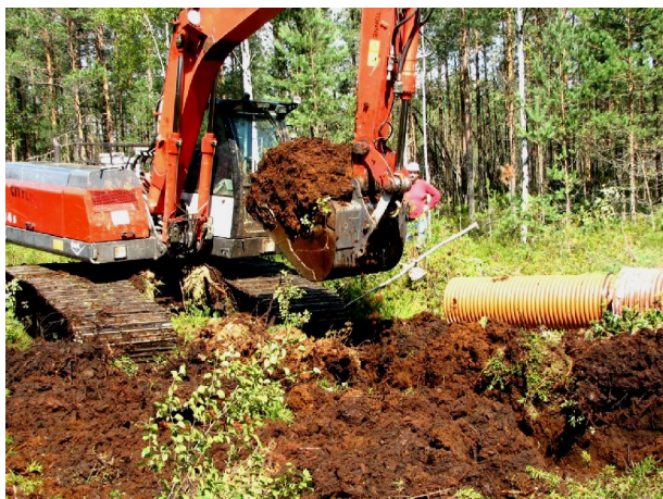
Building of peat dam in Rozu Mire.
