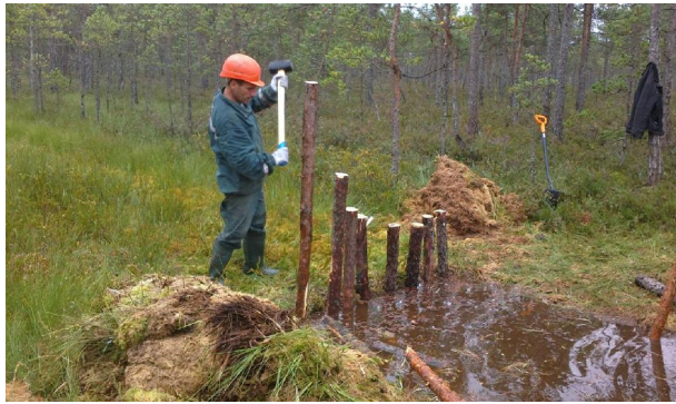
Building of peat/wood dam by hand in Aizkraukle Mire on 03.09.2012. Photo: Arnis Staris
