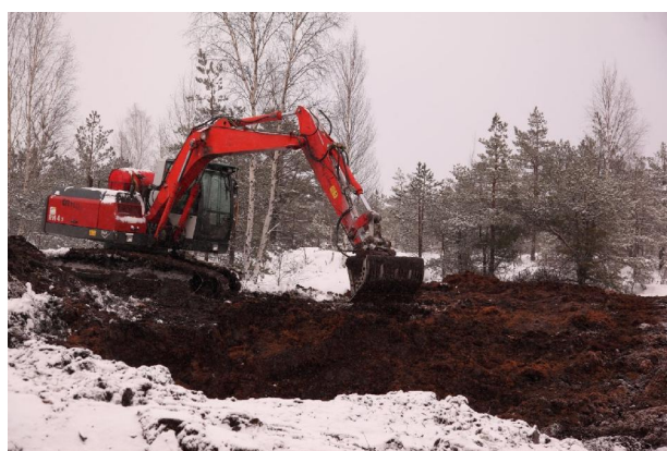
Building of dams in Melnais Lake Mire.
