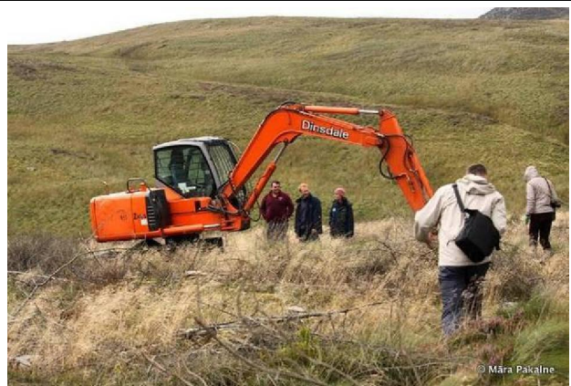
Building of dams in LIFE project site - the blanket bogs in Wales Photo: Mara Pakalne
